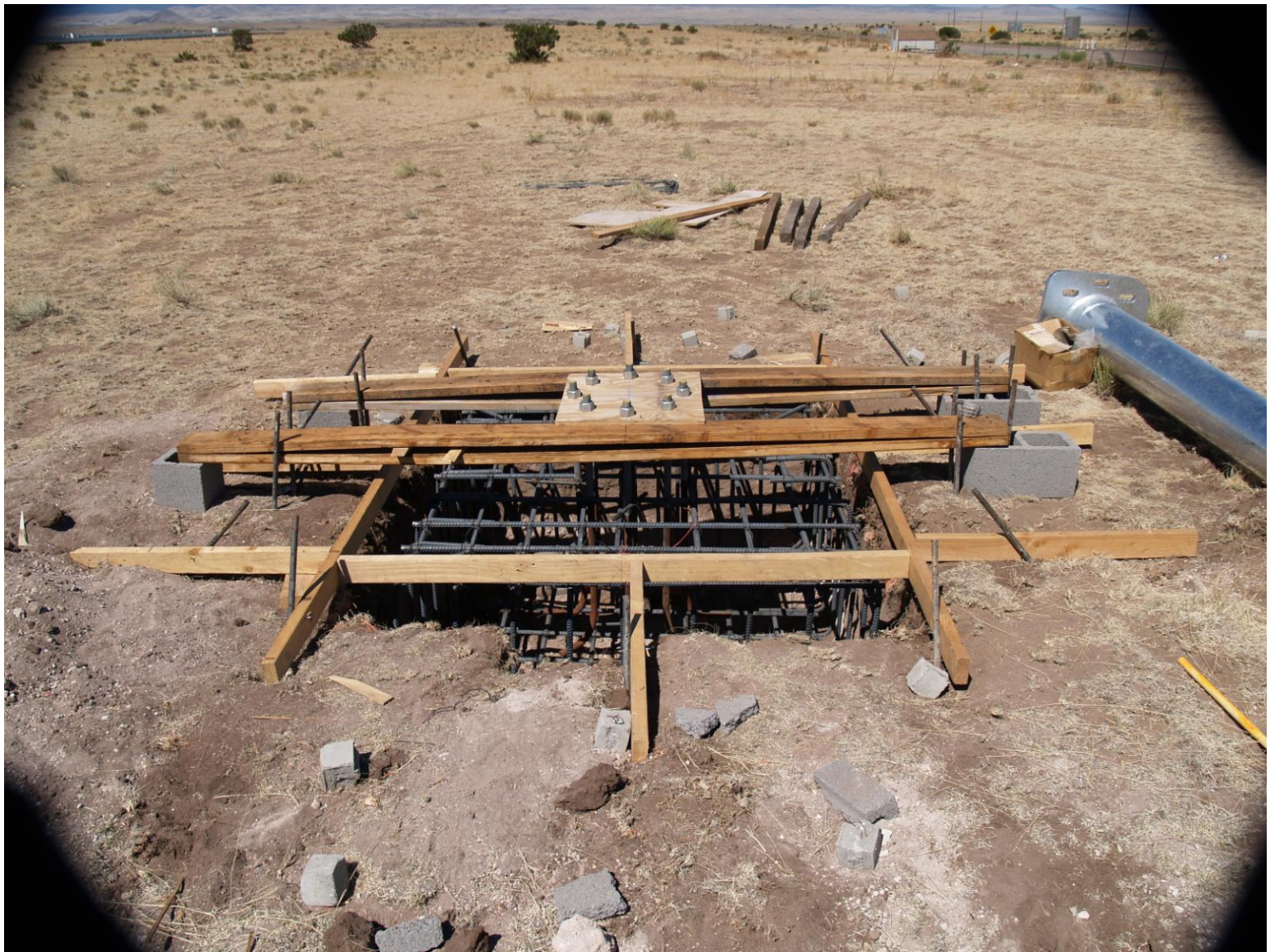
Mat Foundation: 6' x 6' square with a depth of 3'
