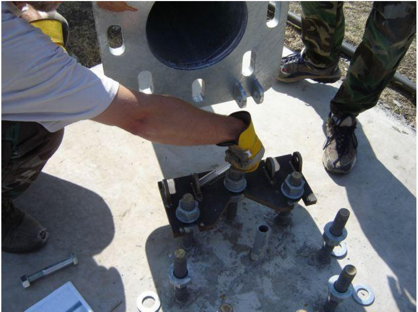
Connecting Tower to Hinge Plate
