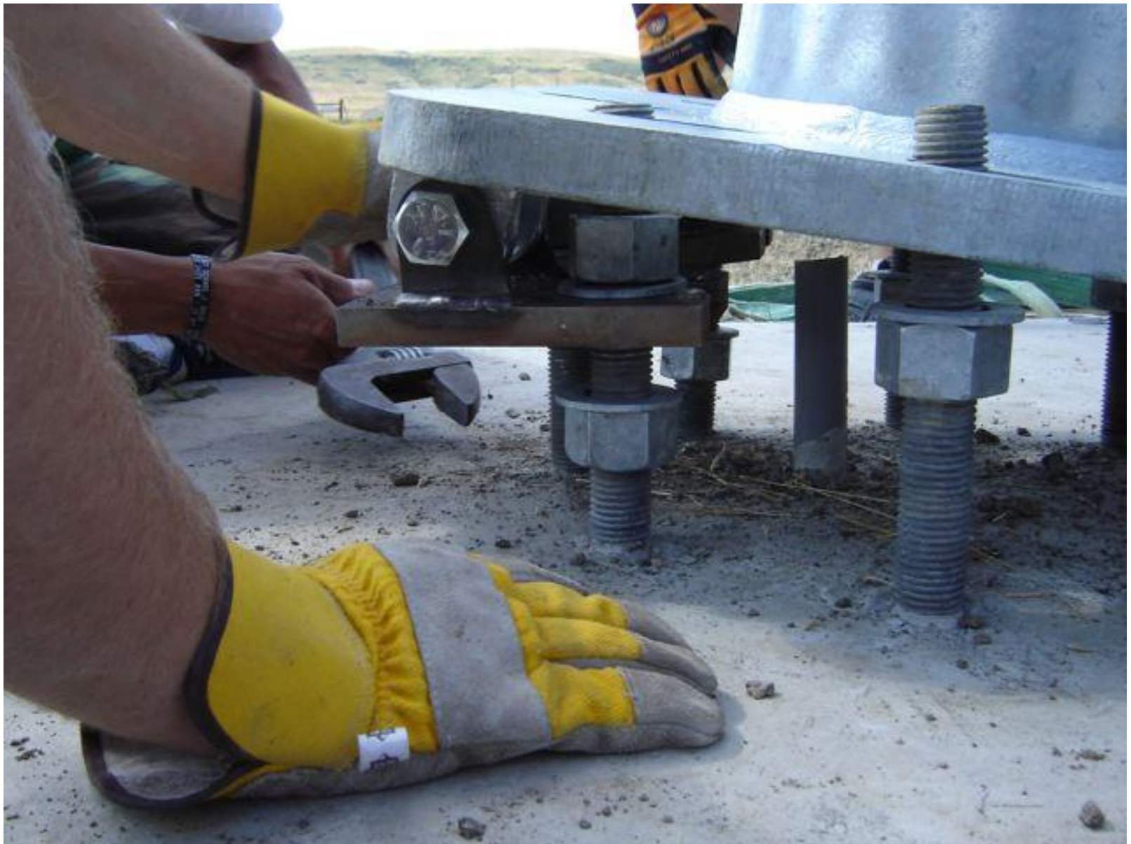
Removing Hinge Plate
