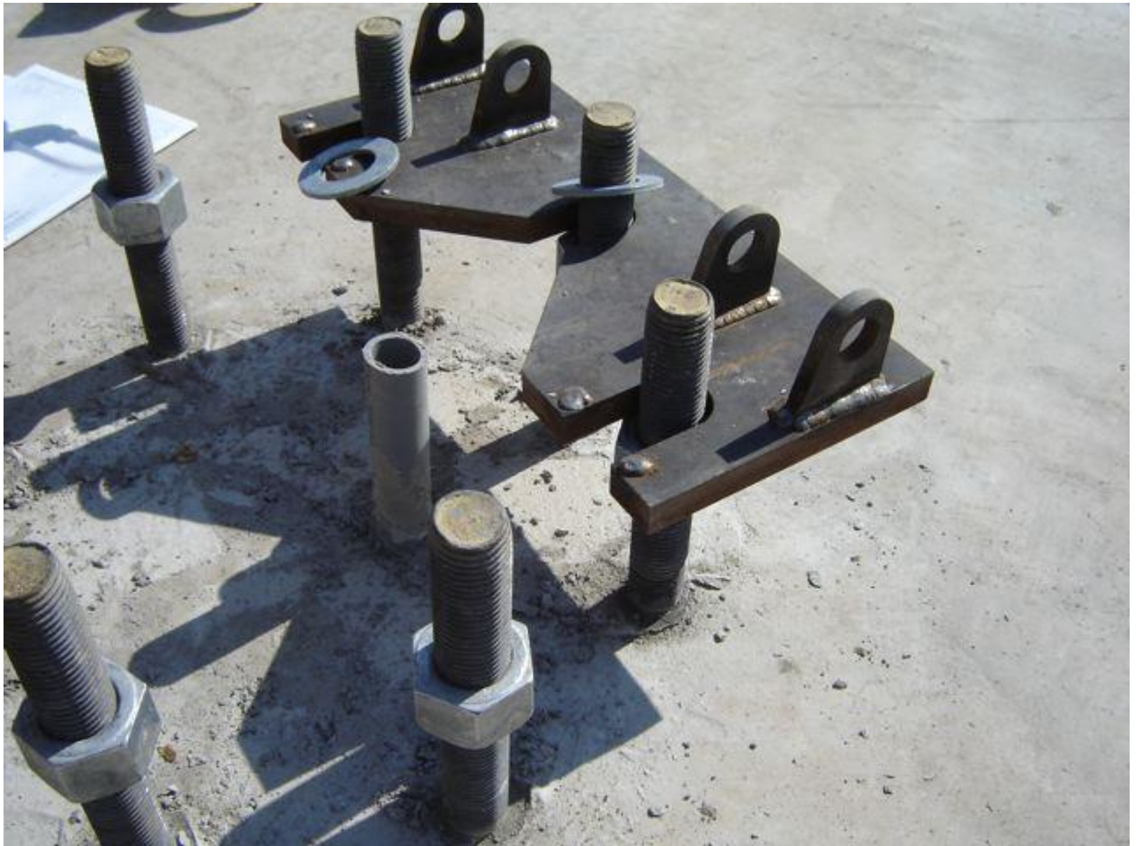
Installing Hinge Plate
