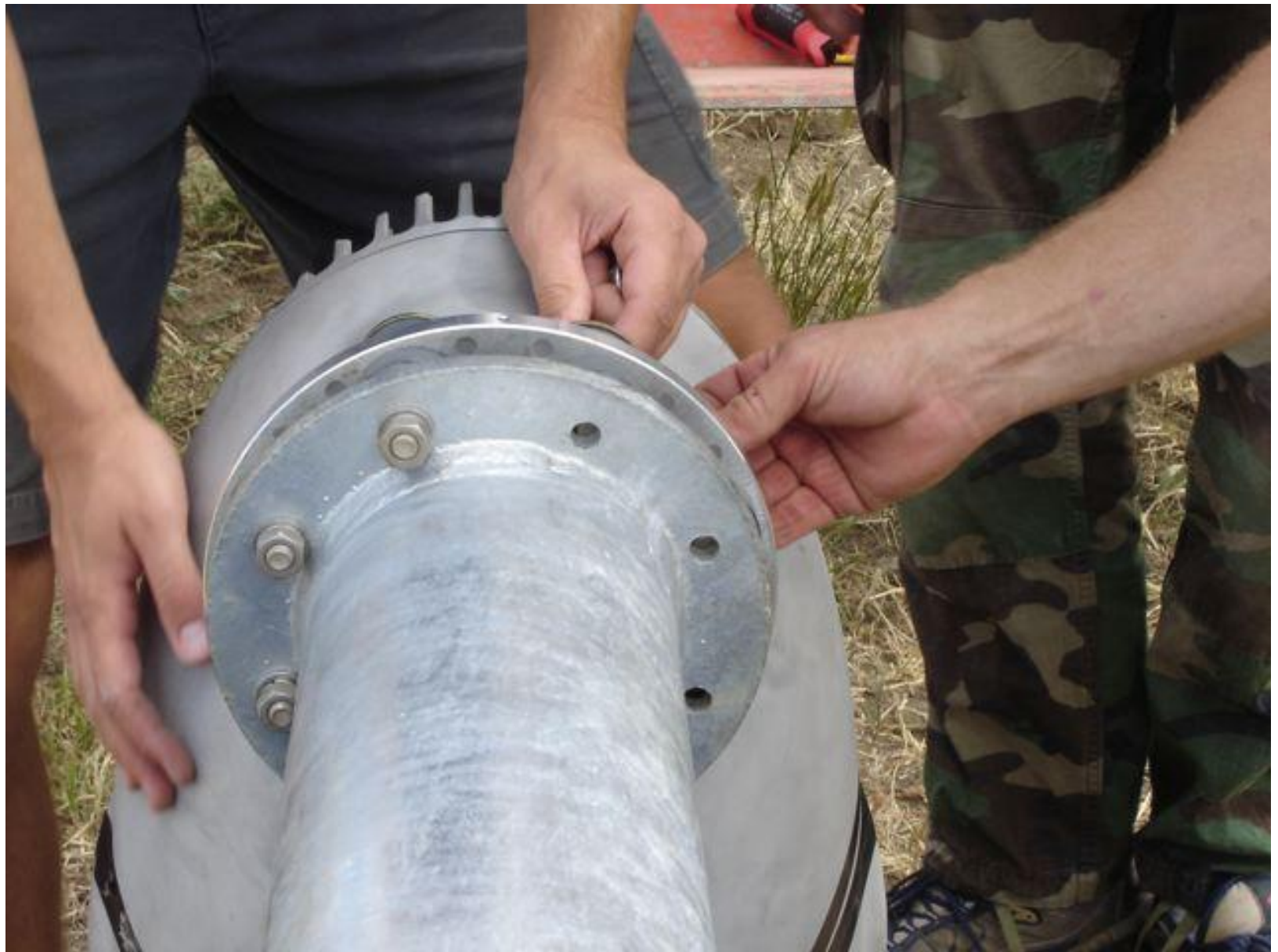
Tighten the Bolts
