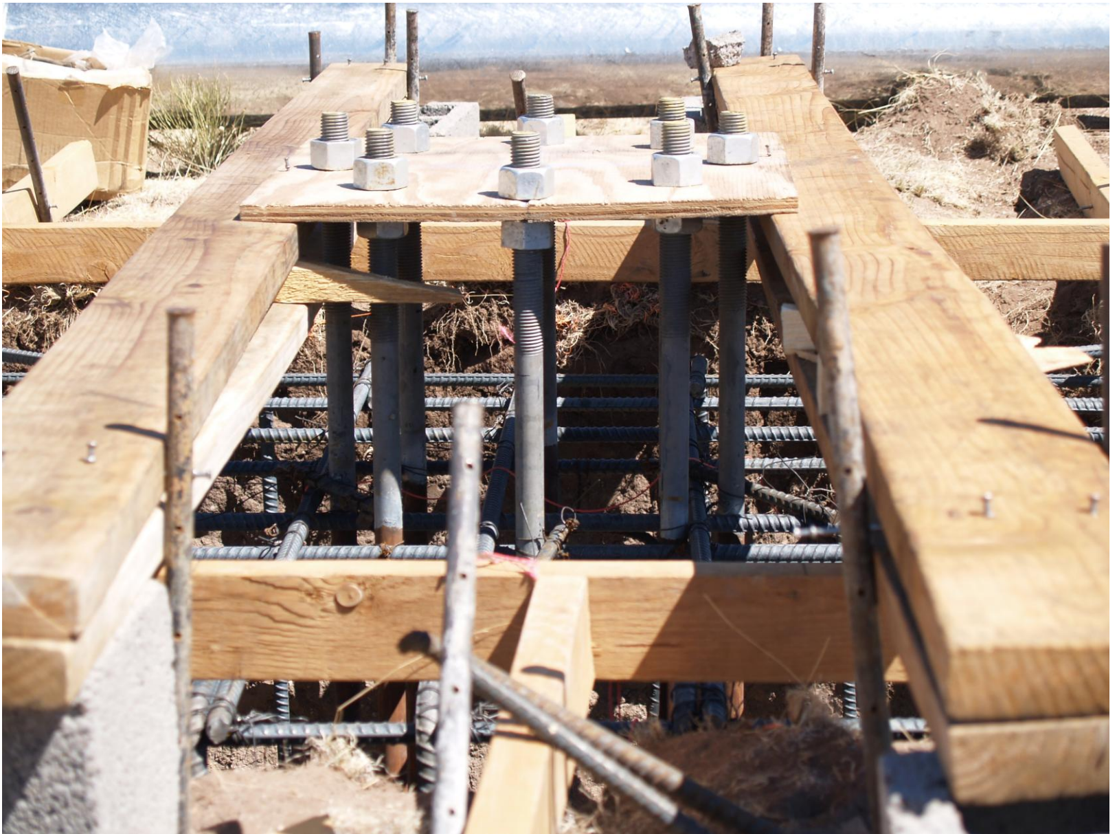
“J” Bolts securely locked in position
