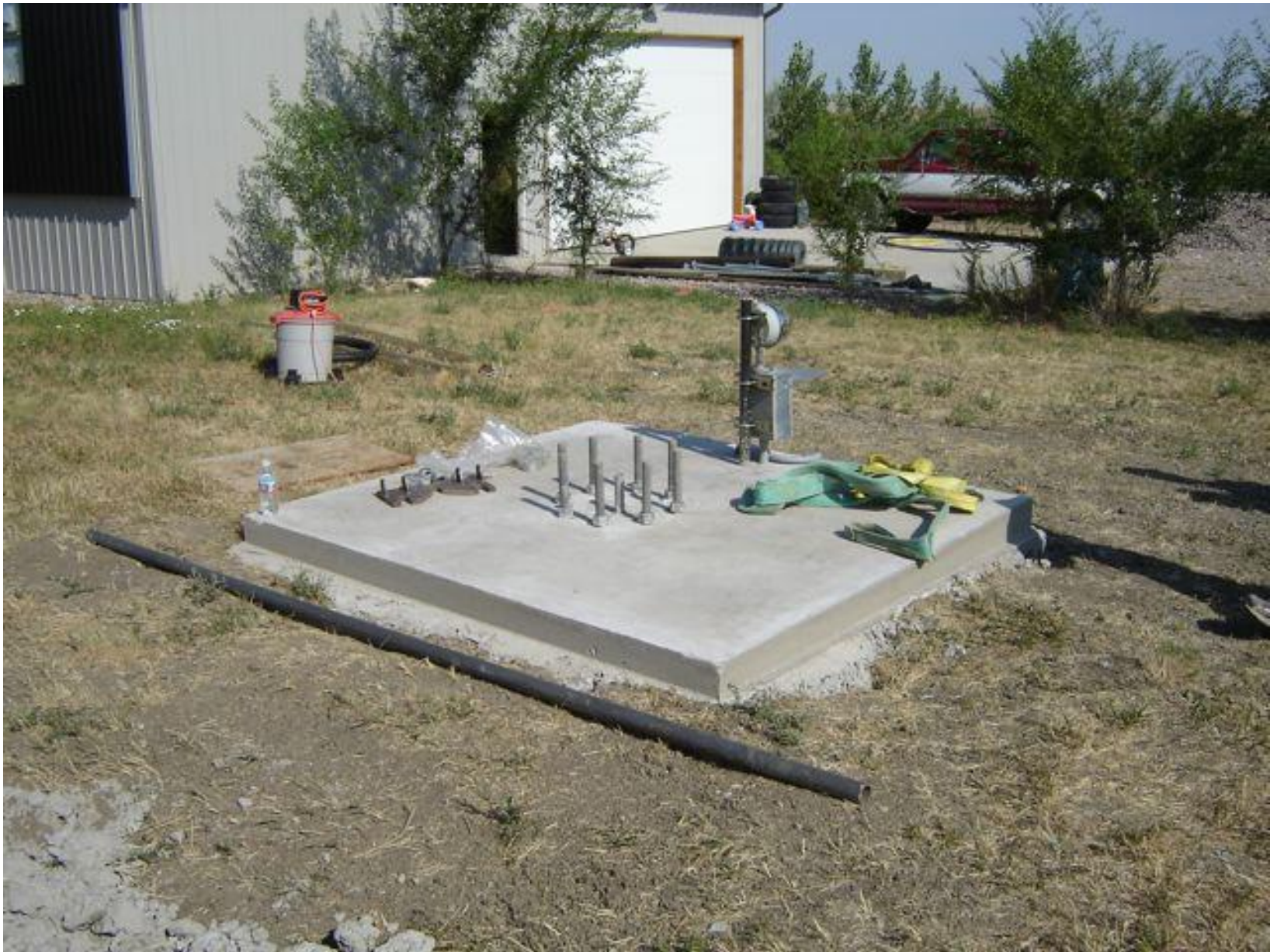
Mat Foundation and Junction Box
