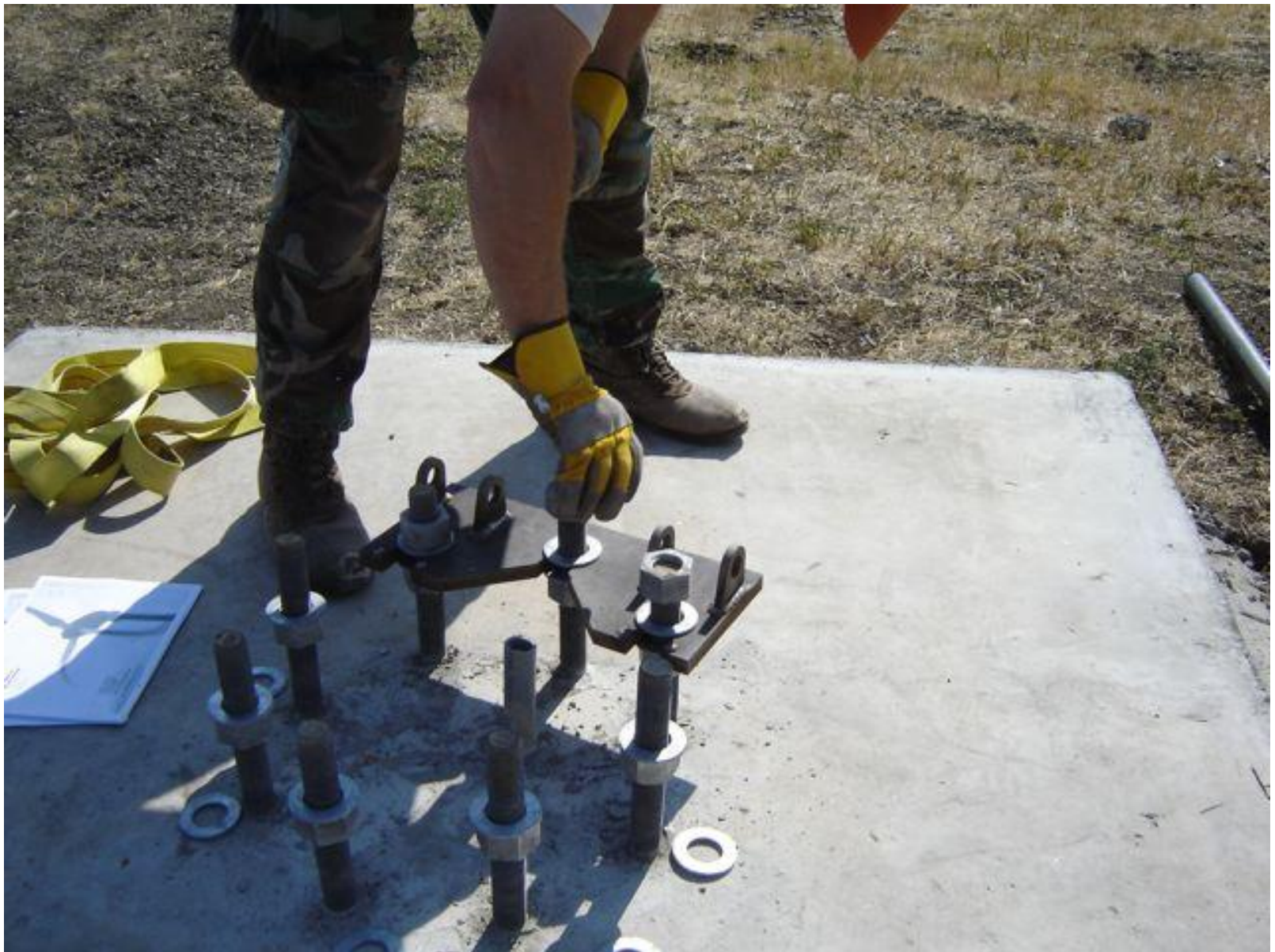
Tighten the Hinge Plate Nuts
