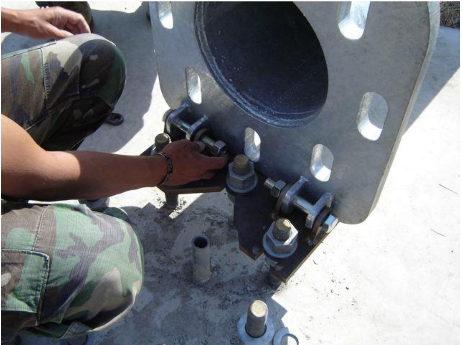
Tighten Bolts and Nuts
